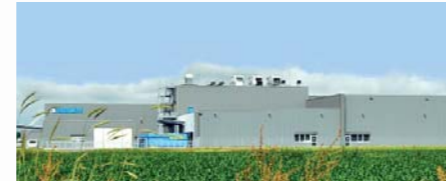
Endingen a. K.: Clean room production according to GMP C + D
